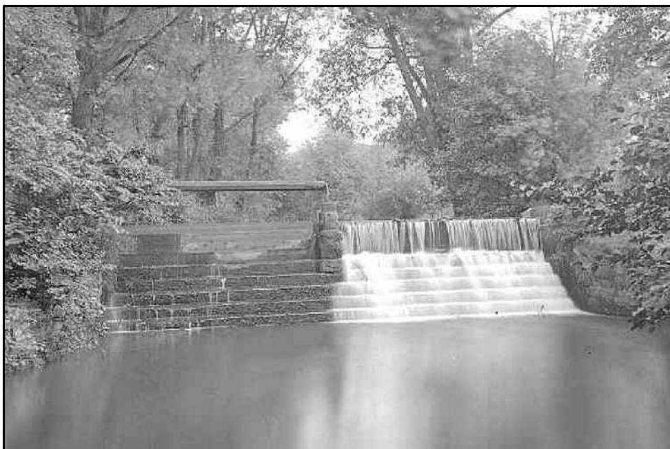
The Dam, photographed in 1936 after completion of a rebuild and overhaul of mechanism. The hydro-generator would still have been operational in 1936, if only as a standby for the diesel.
